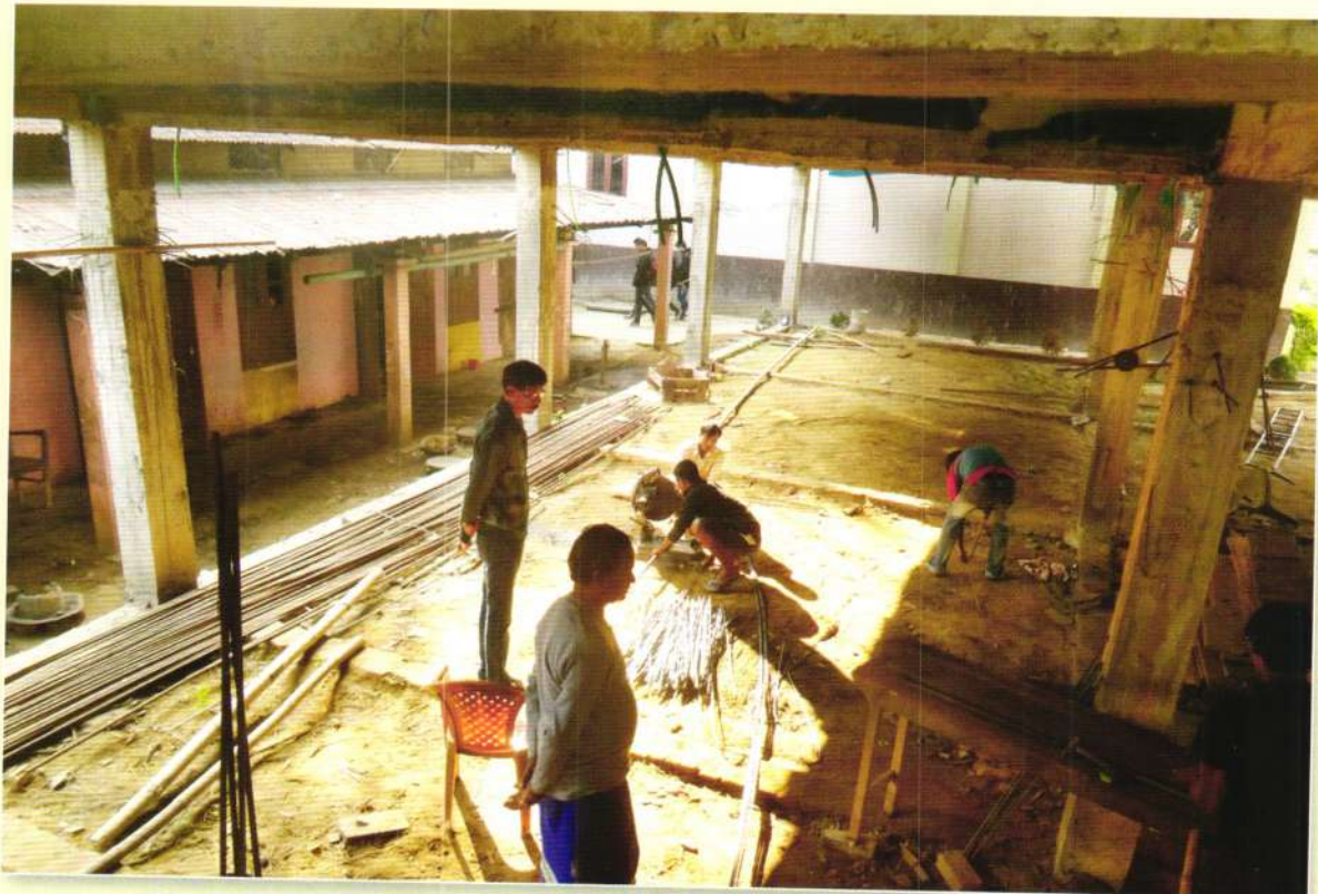
A glimpse from the construction of the new administrative building
